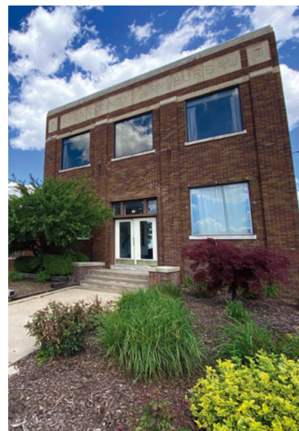
In February, the Knox-Galesburg Symphony in Illinois announced that it is renovating a former Farm Bureau Building, with a goal of expanding music education.
