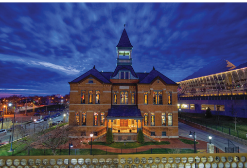
The Webster School building will become the new headquarters of the Kansas City Symphony.
